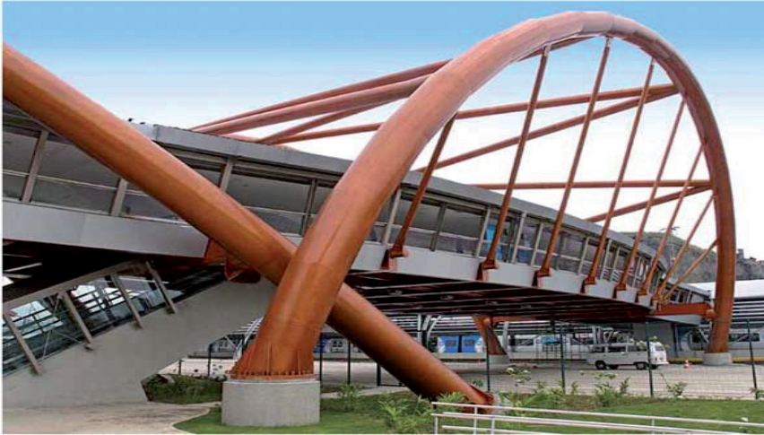
Figure 1. Example of a tubular steel pedestrian footbridge in Rio de Janeiro/RJ, Brazil.
