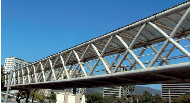
Figure 7. Investigated steel-concrete composite tubular footbridge.
